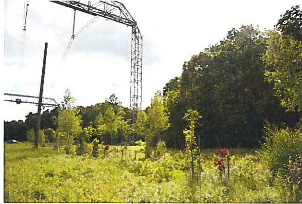
Figure 2-7 Image of the planted trees under the UHV span which were utilized for the natural vegetation withstand tests.
