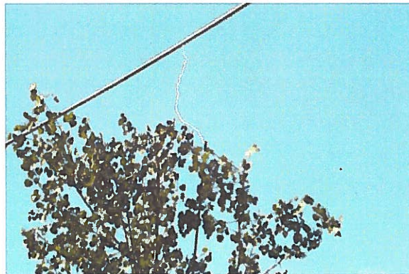
Figure 3-6 Example of a flashover to the cut tree with grounded metal rod.
